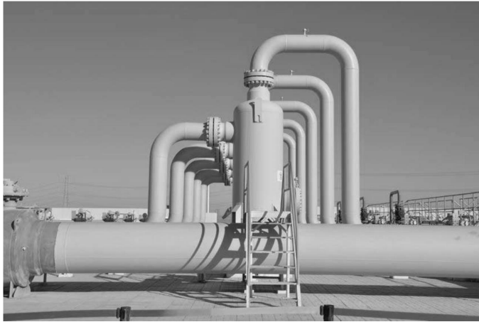
Fig. 1. The actual laying of natural gas transmission pipelines
